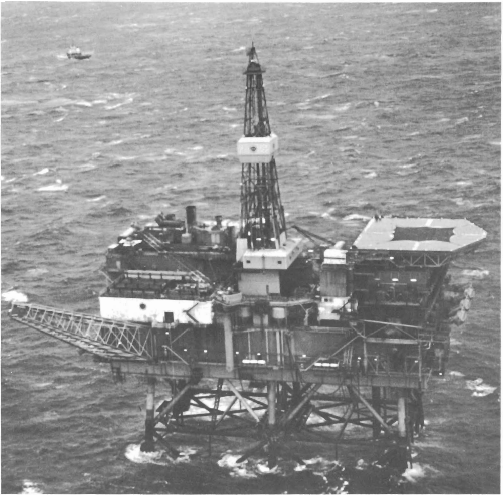
FIGURE 7.8 Brent A platform. (By courtesy of Shell U.K. Ltd.)
