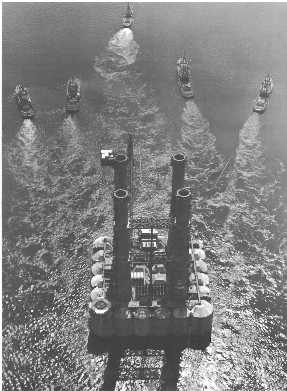
FIGURE 7.10 The substructure of Brent C platform being towed out from Ardyne Point on the west coast of Scotland. (By courtesy of Shell U.K. Ltd.)
