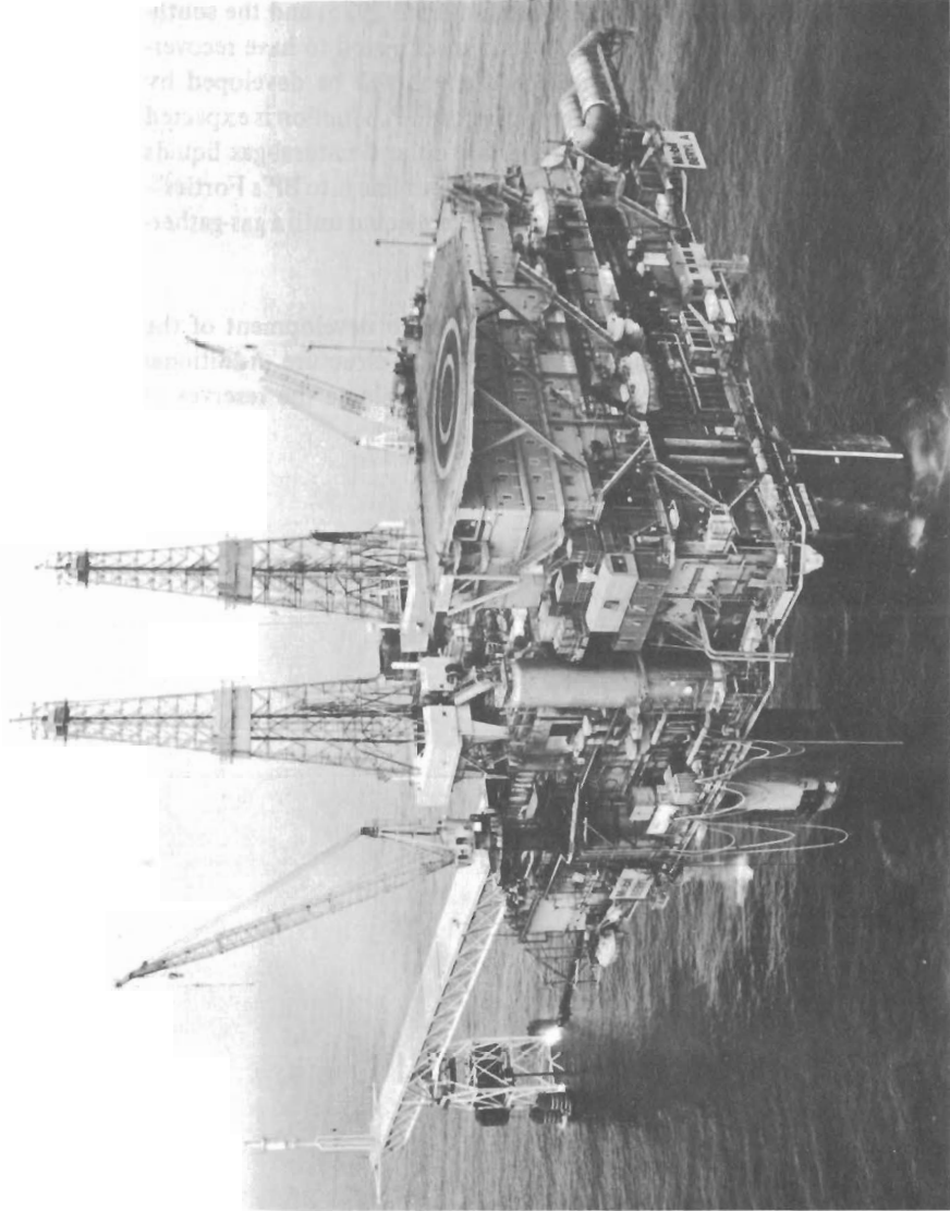
FIGURE 7.5 Beryl A platform. (By courtesy of Mobil Producing North Sea Ltd.)
