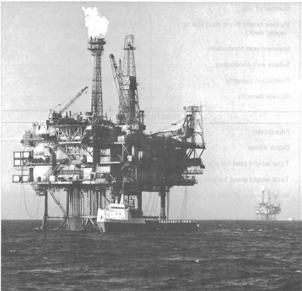
FIGURE 7.18 Forties FB platform (Graythorp II). (By courtesy of British Petroleum.)
