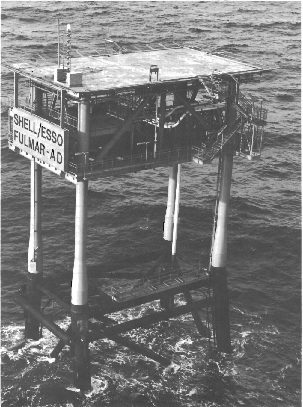
FIGURE 7.21 The substructure and deck of Fulmar well-head platform (B). (By courtesy of Shell Oil.)
