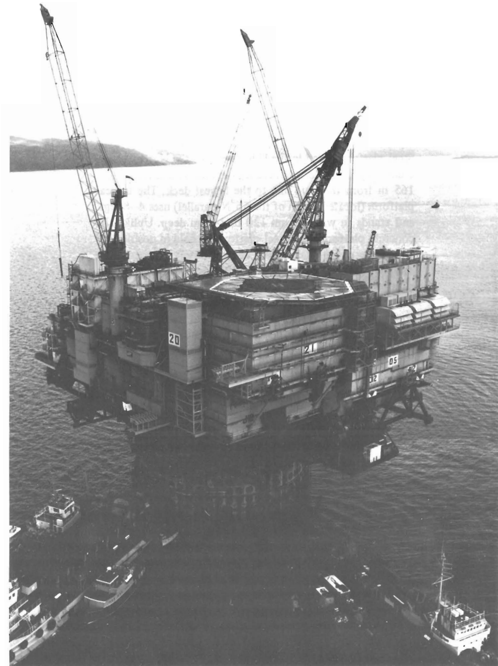
FIGURE 6.4 The largest concrete platform in the U.K. sector of the North Sea: Ninian Central. (By courtesy of Chevron Petroleum Ltd.)
