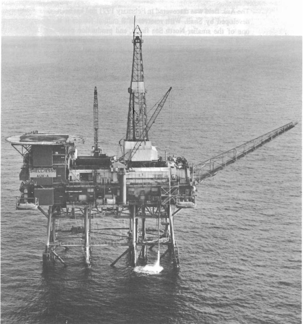
FIGURE 7.2 Auk production platform. (By courtesy of Shell U.K. Ltd.)
