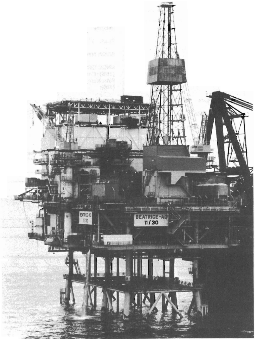
FIGURE 7.3 Beatrice drilling platform. (By courtesy of BNOOC.)
