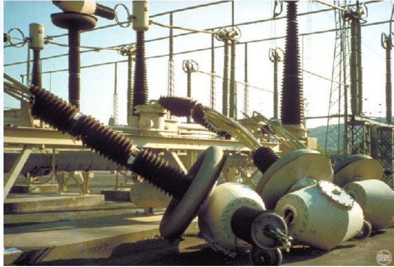
Effects of flooding on distribution station and pylons
