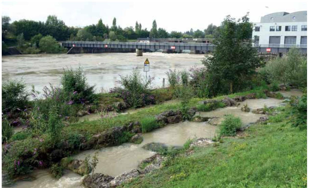
Example of a specific connectivity measure: fish ladder near Olten in the Canton of Solothurn (Switzerland).
