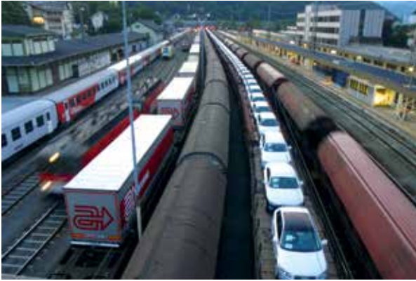
Rail infrastructure along the large Alpine valleys.
