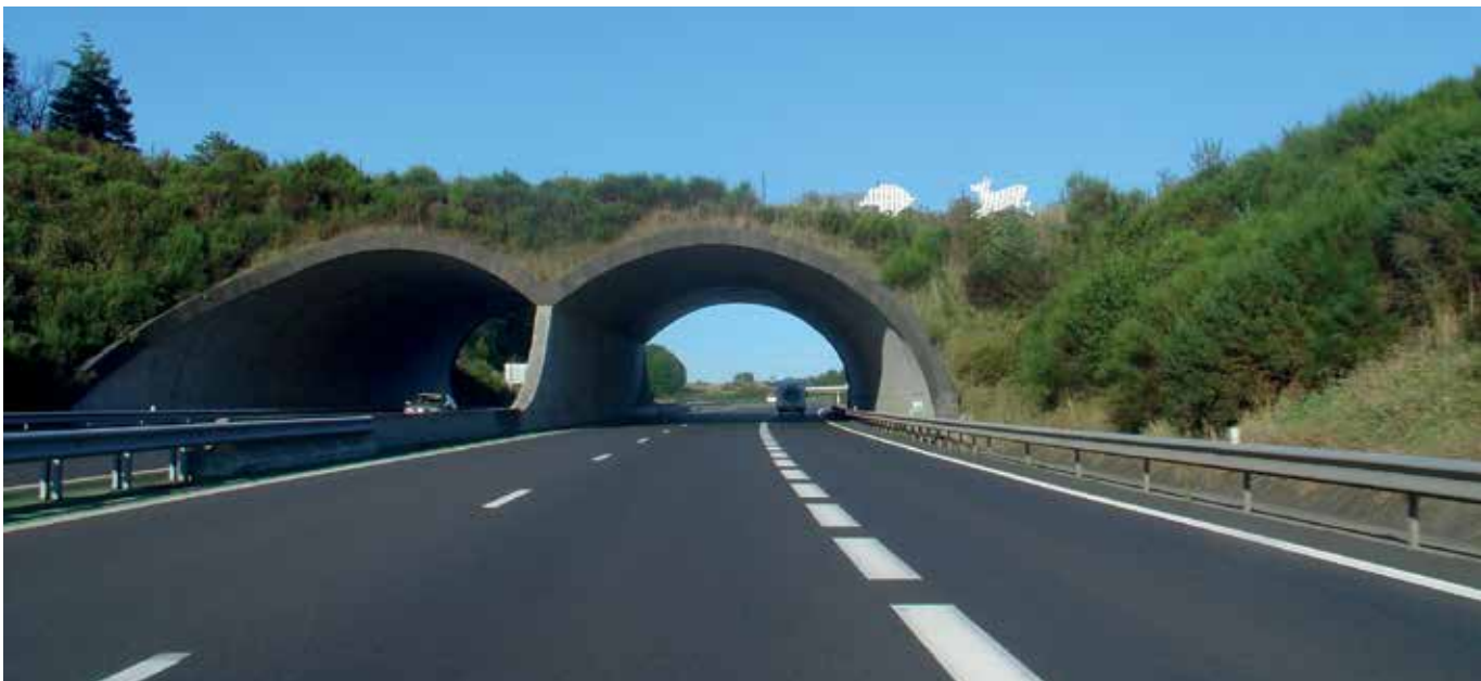
Green bridge on French highway.
