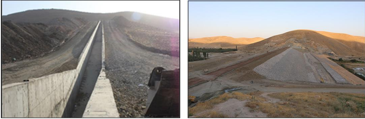
Figure 5-16 Right Jaldian channel to transfer water from Zaab Basin to Urmia Basin. Left Chaparabad dam which is supposed to keep the transferred water from Zaab and release it in none irrigation season to reach the lake. © Somayeh Shadkam
