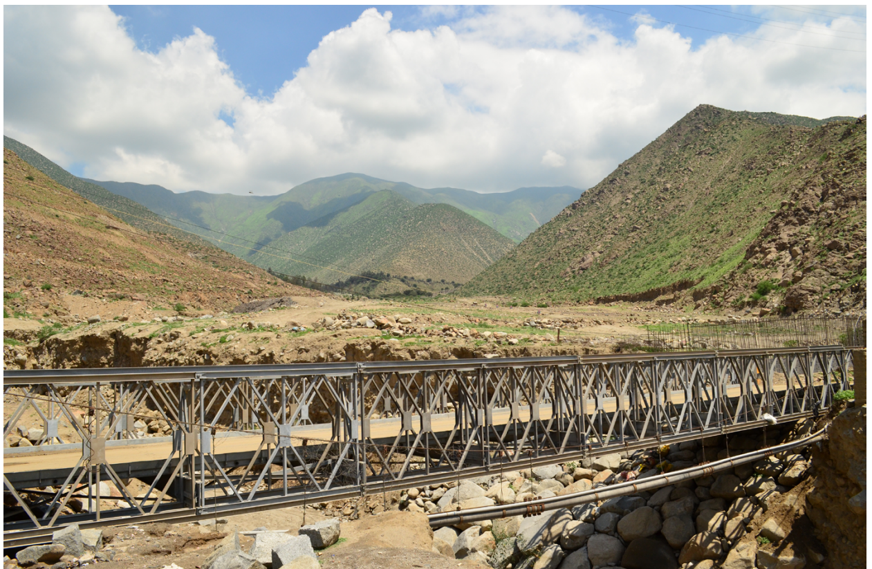
Photo 7: A Bailey bridge established in the wake of the 2017 coastal El Niño.
