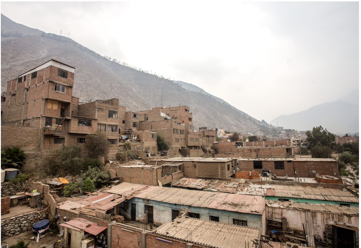
Photo 3: Typical brick and mortar construction in the Rimac River valley.
