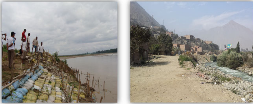
Fig. 17.3 Flood risk context in the Karnali river basin in Nepal (left panel) and the Rimac river valley in Peru (right panel). Photo Sources Practical Action and A. Keating
