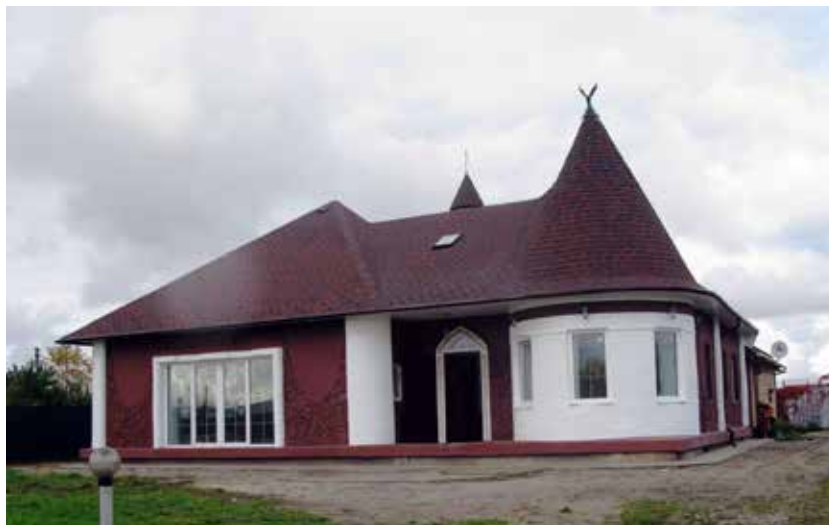
Figure 40. The first residential building in Europe printed with a 3D construction printer. Yaroslavl (Russia). Source: AMT-SPETSAVIA Group (Russia) – www.specavia.pro , CC BY-SA 4.0, https://commons.wikimedia.org/w/index.php?curid=74334750 .
