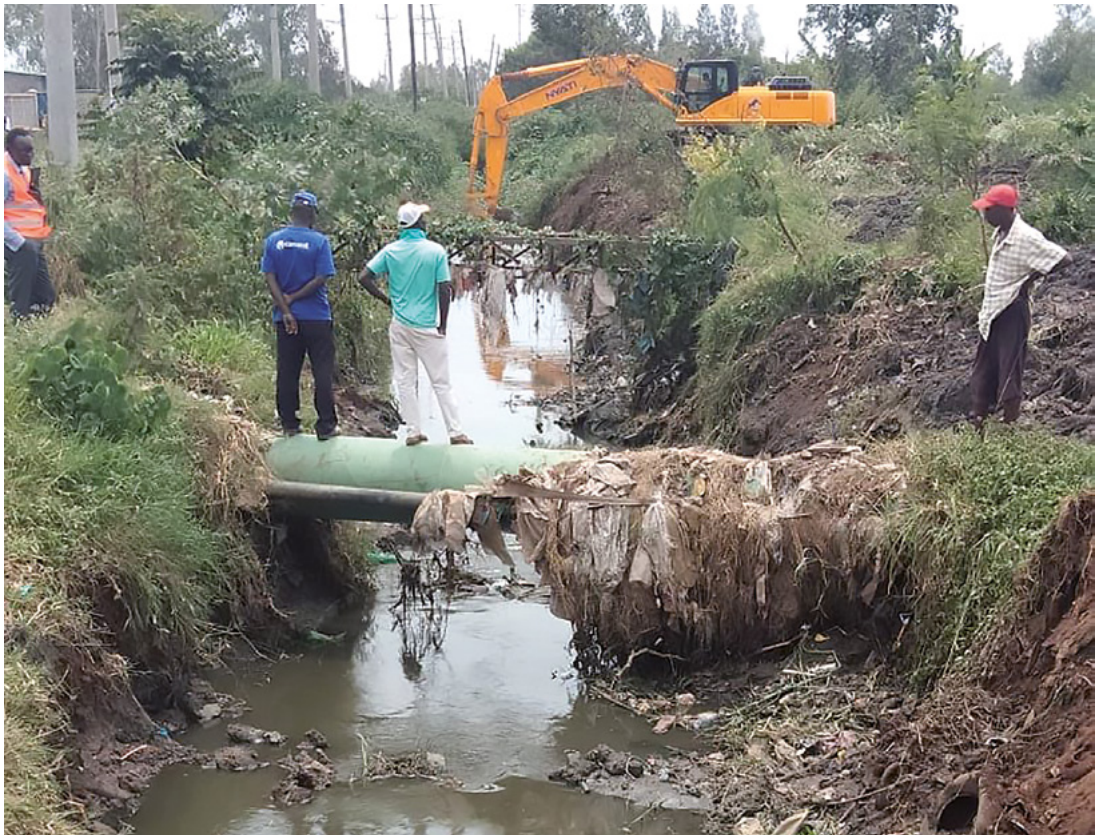
Clean up work in Kisumu, Kenya (Source: Tejas Patnaik /UNDRR)
