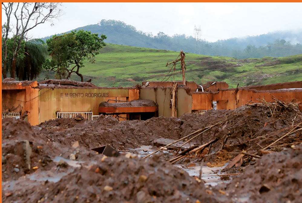
Debris and damage at a school in Bento Rodrigues, Brazil from the upstream dam failure (Source: Rogério Alves/TV Senado 2017)
