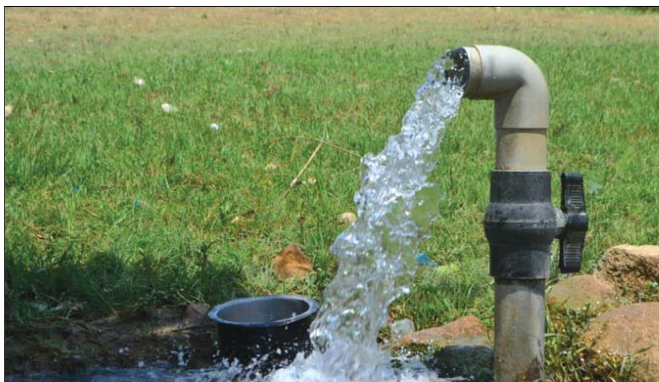
A tube well built under PIM
