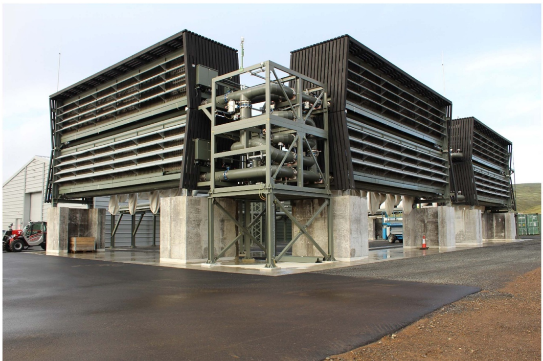
Figure 3. The Climeworks 4000 tons yr -1 demonstration DACCS project in Iceland. Source: Authors, during a site visit to ON Power's Hellisheiði Geothermal Power Plant in September 2021.
