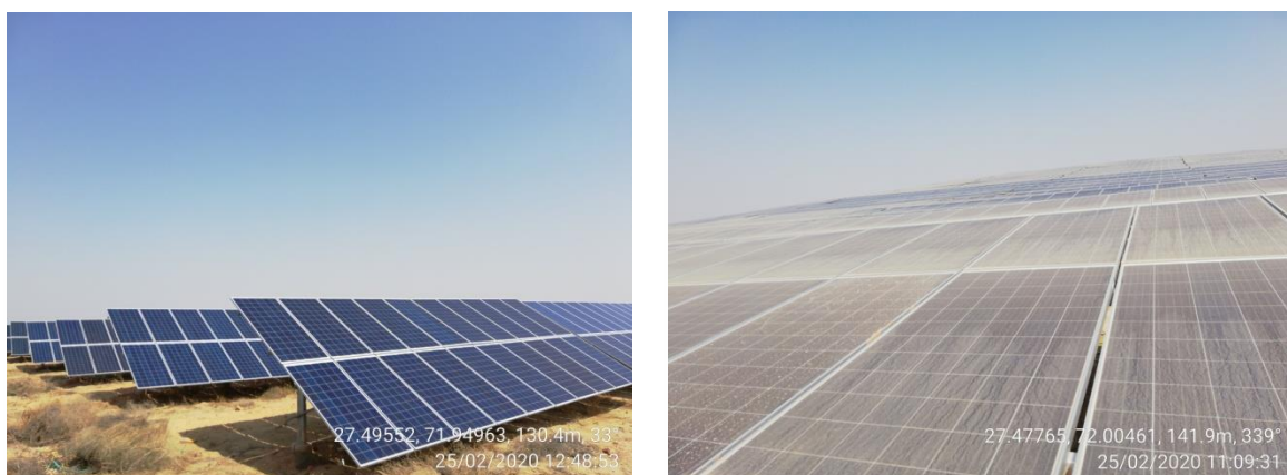
Figure 4. (a) Photographs showing the photovoltaic solar panels during the clean condition and (b) during the sandy deposition stage in the Bhadla Solar Park, Jodhpur District, Rajasthan State, India.
