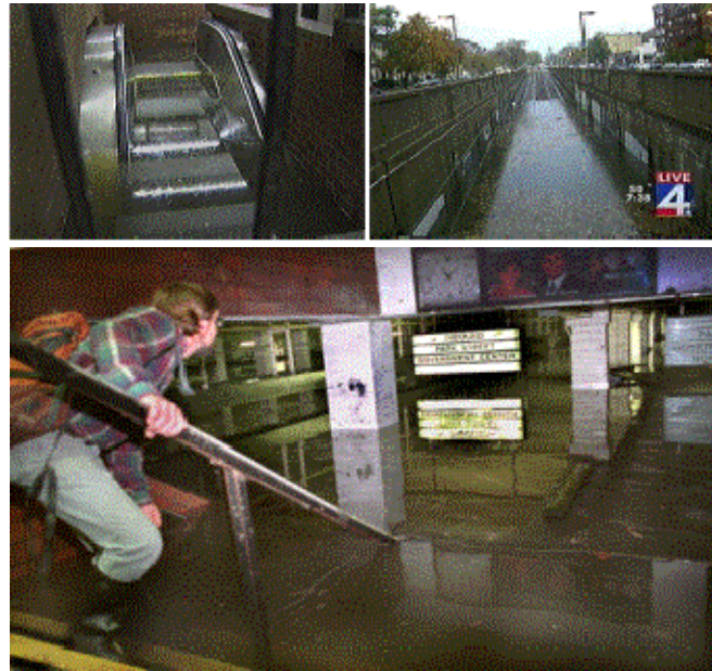
Figure 4.1: Images from flooded Kenmore Square Station. Photo Credits: WBZ-TV/CBS, WLVI-TV/WB, John Tlumacki (Boston Globe)
