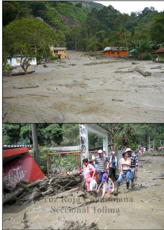
Figure 2. Recent landslide disasters in the Combeima valley: upper picture: houses destroyed and severely affected by the July 2009 landslide in Villa Restrepo; lower picture: local people after the similarly destructive landslide in June 2006 at the same location (photo courtesy of the Tolima Regional Disaster Prevention Committee and the Colombian Red Cross).
